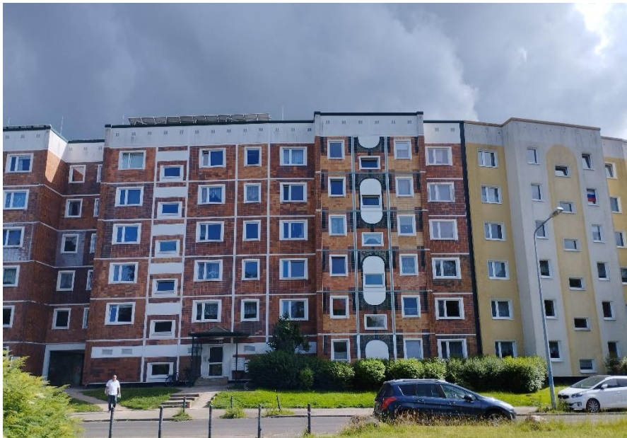
Figure 16: Housing in the outer parts of G5
